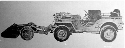
Jeep-mounted mine detector, AN/VRS-1, produced by EMR for The Engineer Board (*History* of the Development of Electronic Equipment - I - Metallic Mine Detectors, The Engineer Board, U.S. Army Corps of Engineers, 1945).
